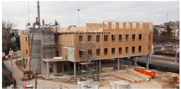
Leake Hall - A Type V Podium Building Under Construction Client: MICA
