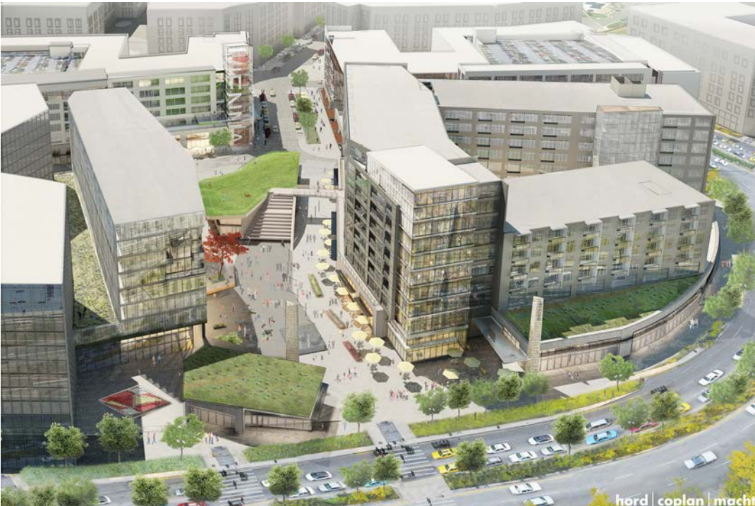
This perspective shows a mix of uses including a Wrapper Building in the upper right. The design calls for market rate apartments around a parking structure with ground-floor retail space. The image depicts the plaza between the buildings with a wrapper building beyond.
