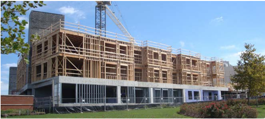
Crosswinds at Annapolis Town Centre - A Type V Podium Building Under Construction, described as Option 1 Client: The Bozzuto Group
