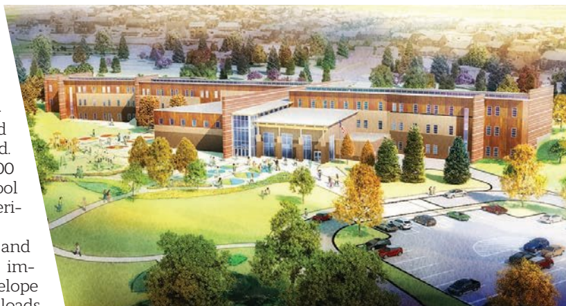
Anthem P-8 is a new preschool through eighth-grade school under construction on a 13-acre site in Anthem Highlands, a planned community of approximately 2,600 residential units, in Broomfield.
