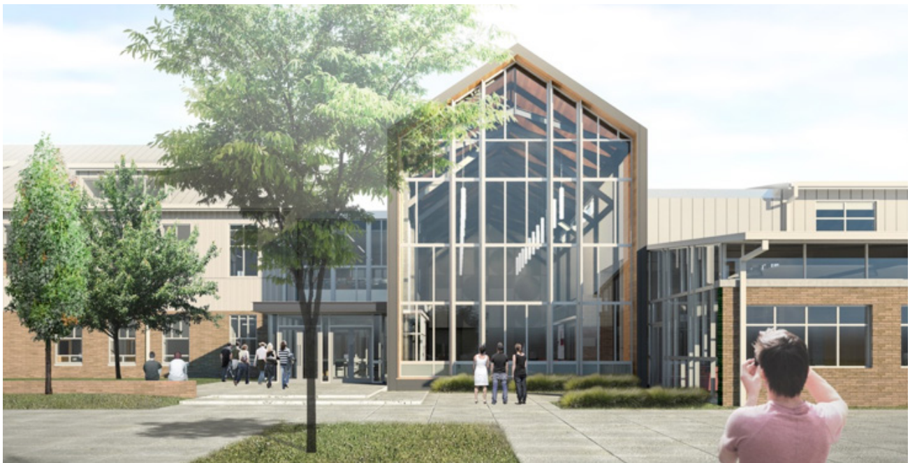
HCM honored the NDHS legacy by repurposing wood from the old school to use in the new structure.
